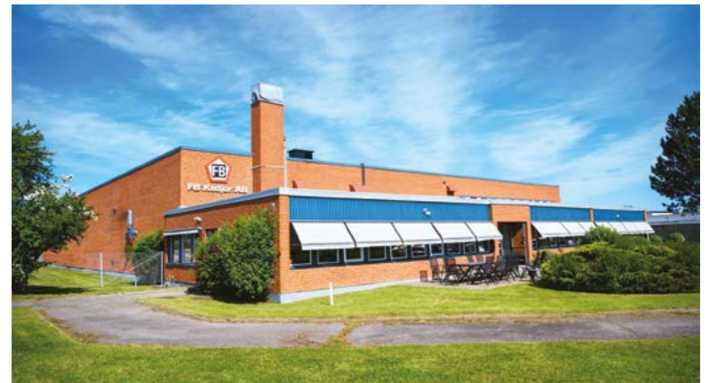
02. FB Kedjor office, warehouse and workshop
